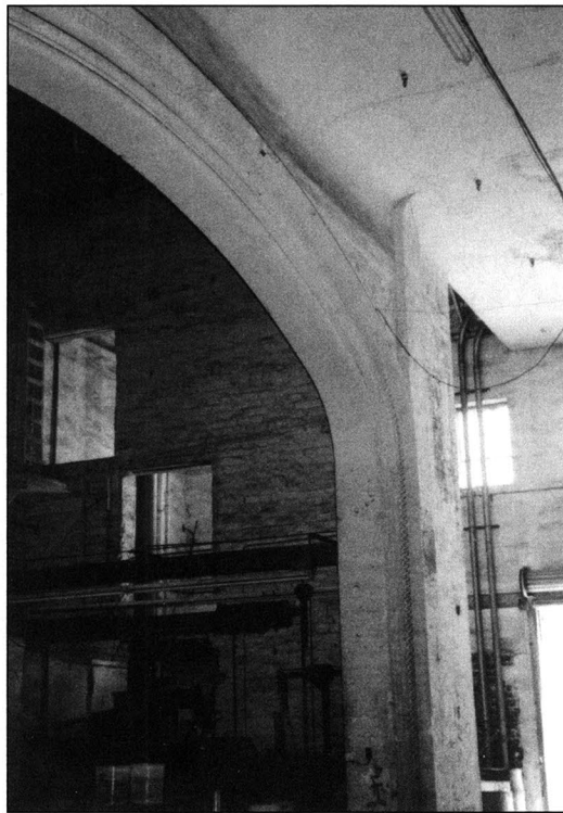
The Rialto Theater, interior view, displaying ornamented plaster proscenium surround. (Photograph courtesy of the author.)
